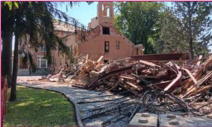
Demolition and debris.
